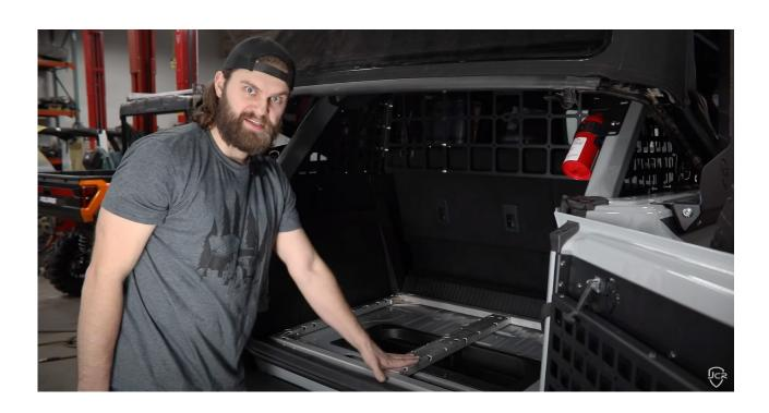
**6.** Now that the frame is in place, take the factory bolts that were removed to hold down the factroy hooks and use them in the same locations to secure the frame to the floor. Using a 10mm socket secure the bolts through the corner support brackets into the factory threaded holes.
